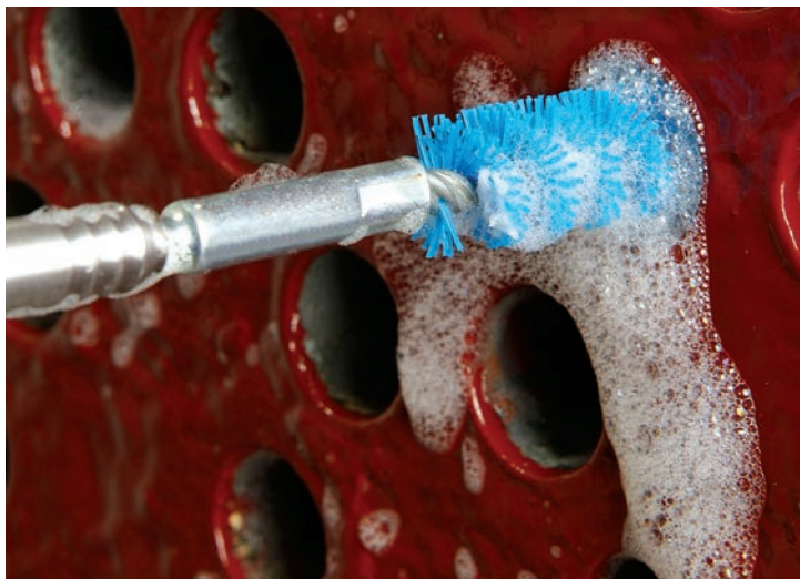
Internally enhanced tube before cleaning with RAM-6.
